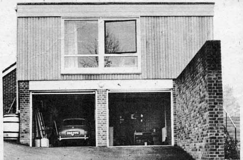
View of large double garage shows how it is built under the sitting-room and hidden from the garden by the brick wall
