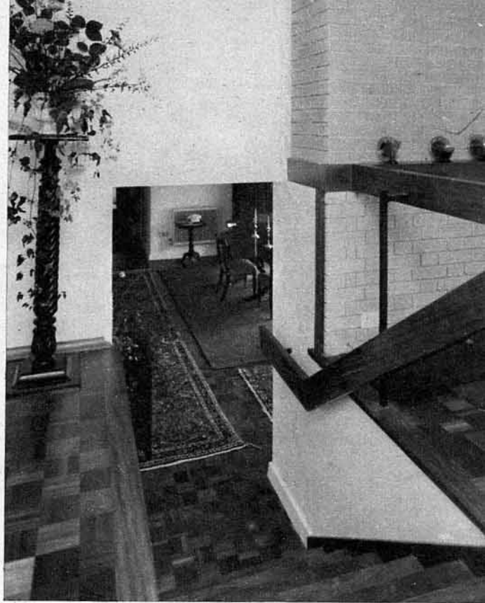
Wooden stairs cope with the different levels of sitting and dining-rooms. Floors are wood block throughout. Central heating is by radiators all over the house except in the sitting-room where there is skirting heating
